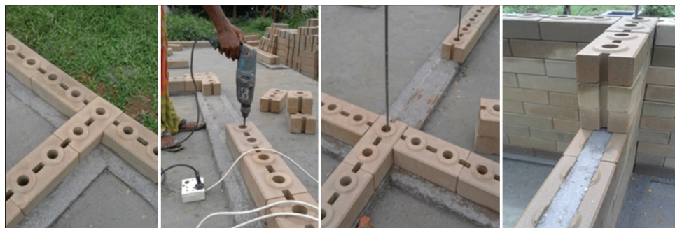
Figure 4: Placement of the first course of bricks
