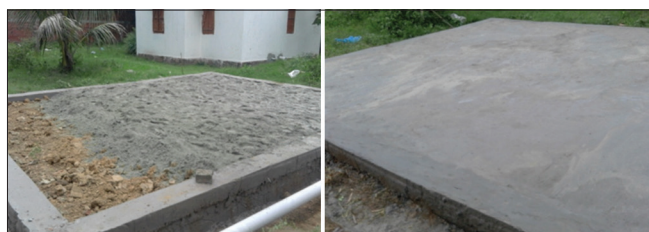
Figure 3: Completion of first-floor area
