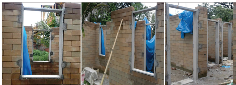
Figure 5: Installation of wooden frames
